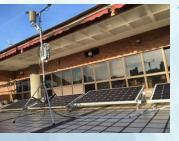
建成了光伏發電及儲能為本智慧型 微電網實驗室,是全港首個先進微 網控制實驗平台,總容量達 4 kw。 A first of its kind microgrid platform in Hong Kong dedicated for scientific experiment and practical implementation of advanced microgrids control algorithms.
