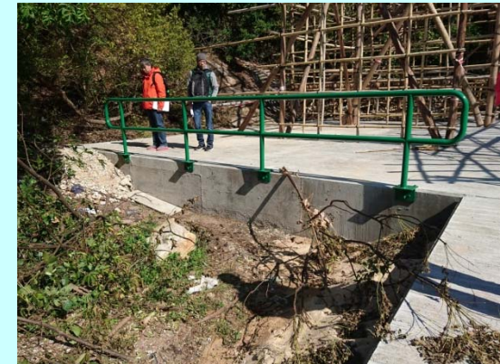
Space near existing platform (Equipment Room)
