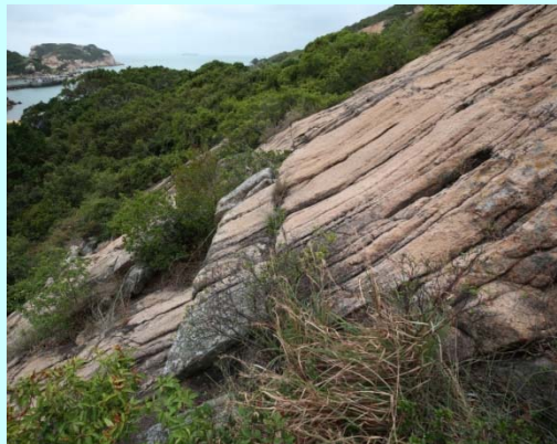
Slope near Aqua Privy (PV Panel)
